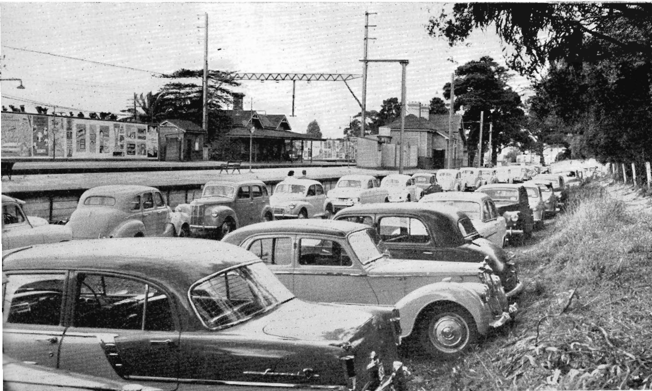
CAR PARK AT CHELTENHAM
